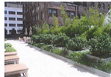
VARIED-HEIGHT PLANTER BOXES ON SUSPENDED SLAB
