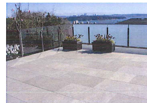
PEDESTAL PAVERS ON SUSPENDED SLAB
