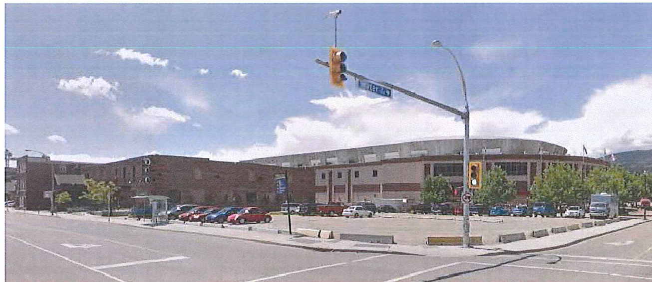
NORTH-EAST CORNER VIEW
