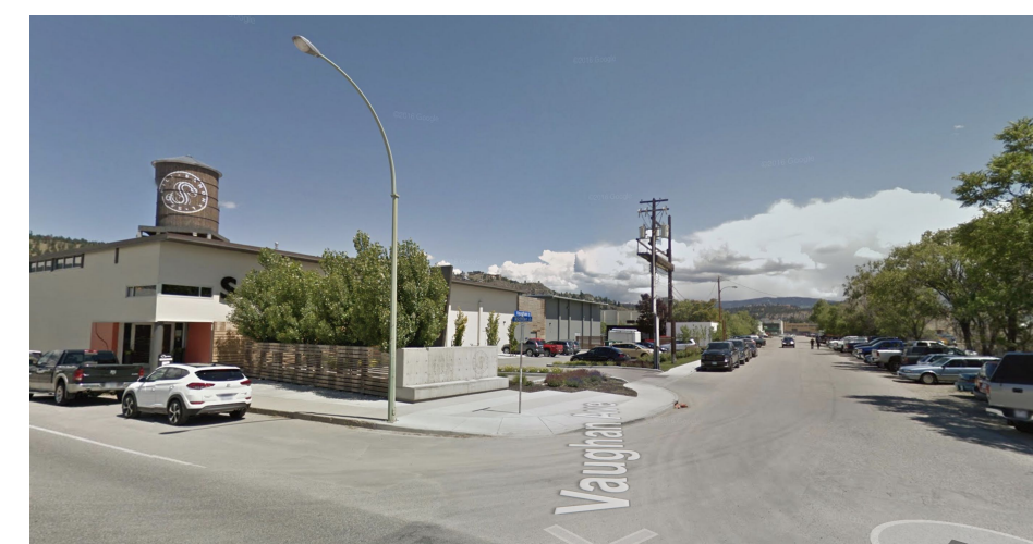
P4: Existing Site view from corner of Vaughan Ave and Richter St looking northeast
