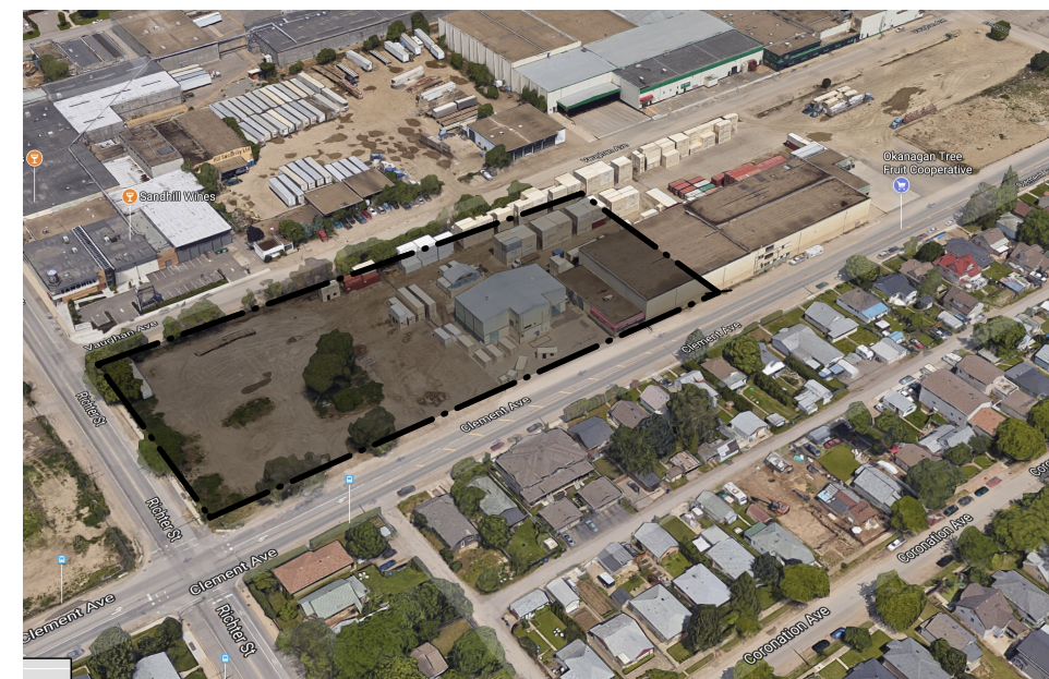
P3: Existing site bird's eye view looking from southwest
