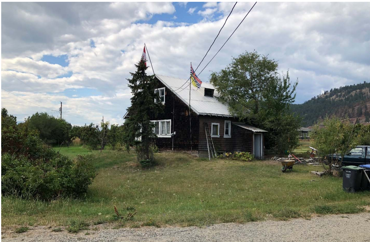
6. Current farm house on site (to be demolished).
