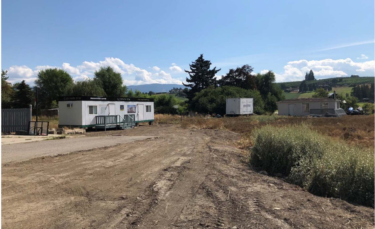
3. View looking east over future road dedication area (Glenpark Drive).
