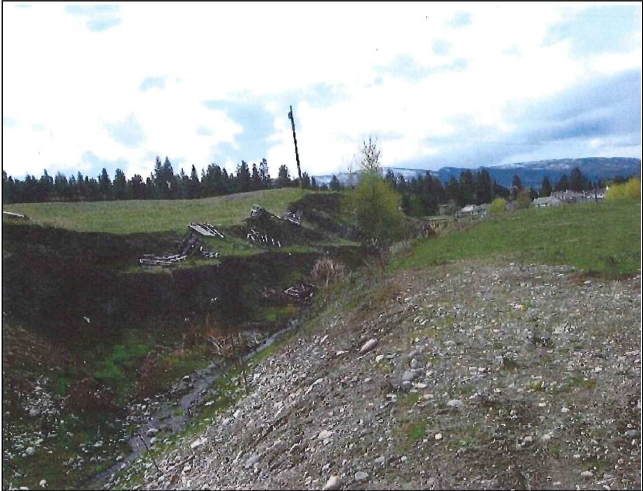
Photo 1 - Canal-channel dug along eastern property boundary as water catchment for SEKID out flow, located near telephone pole in photo, and Ahern Spring.
