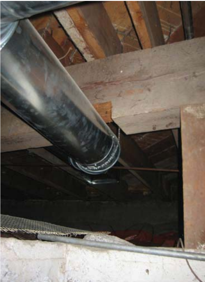
Notching of joist
