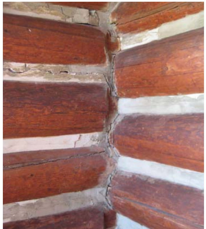
Interior cementitious daubing, front porch
