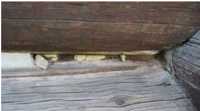
Damaged daubing with chinking exposed to weather, east elevation
