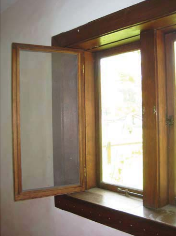
Above: Original window with tapered casing and stool; Top right: Wood window, north elevation; Bottom right: Original front door
