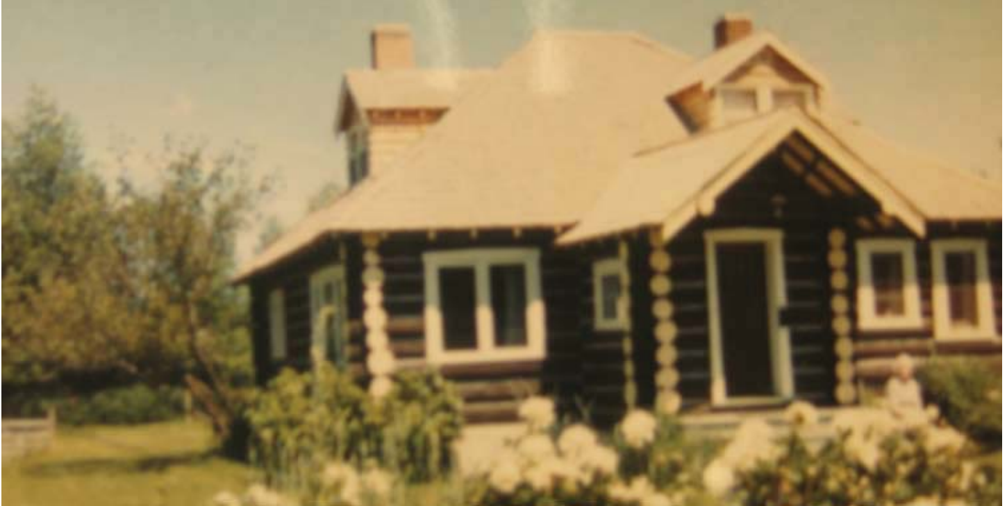
Cameron House, installation of three roof dormers and a new cedar shake roof, before 1968
