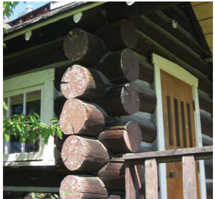
Corner with saddle-notched logs.
