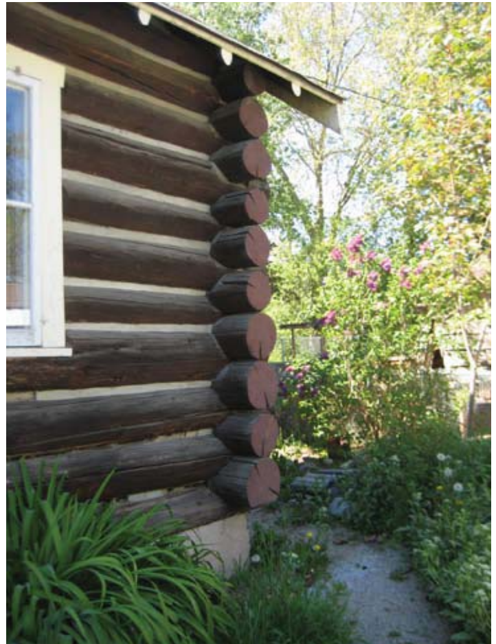
Log construction of east wall.
