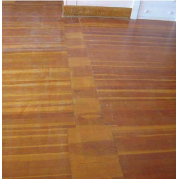
Ghost of removed partition wall
