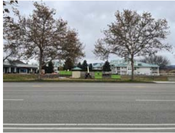
D VIEW FROM GORDON, LOOKING NORTH EAST
