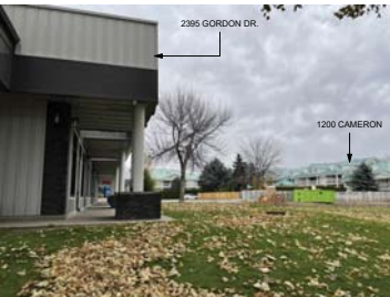
E VIEW FROM GORDON, LOOKING EAST
