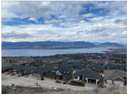
VIEW LOOKING NORTH WEST FROM LOCATION ON SITE NEAR BUILDING 14
