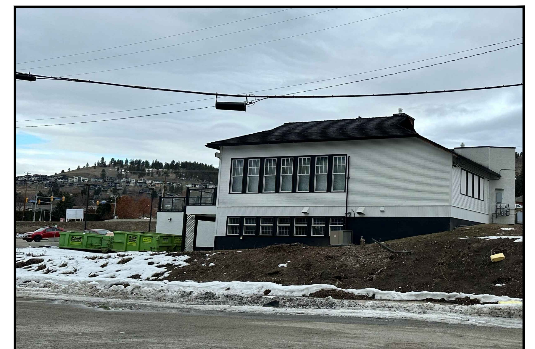
G VIEWING NORTHWEST FROM JOE RICHE RD TOWARDS THE EXISTING SITE
