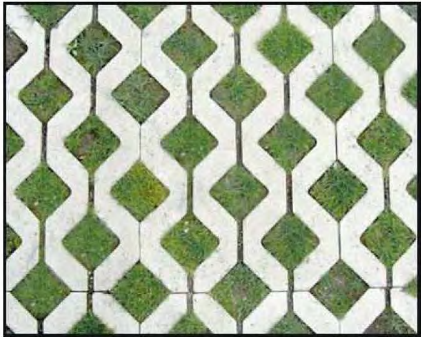
PERMEABLE GROUND WORKS
