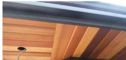
HORIZONTAL SIDING & SOFFIT Clear cedar; stain
