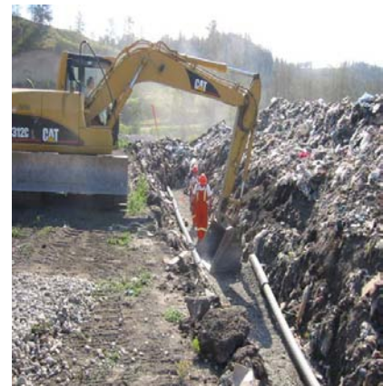
Laying pipe to collect landfill gas at Glenmore Landfill
